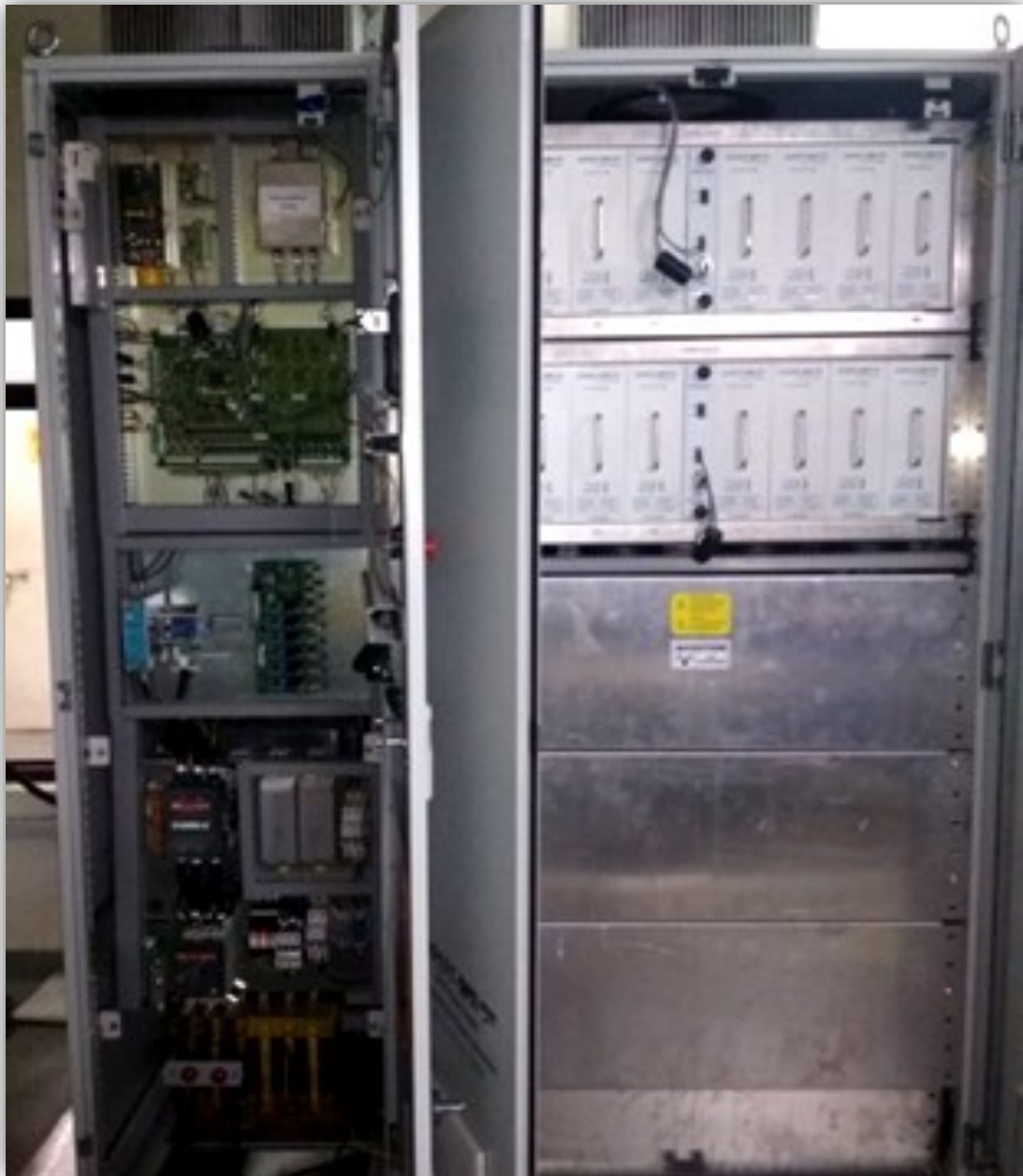
Figure 3: Solid State RF Generator
