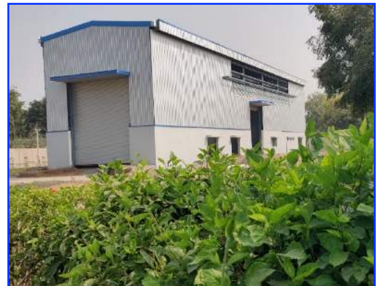
Figure 2: Construction of the housing facility in progress
